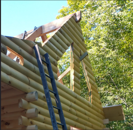
Ridge beam has been set and final gable log pieces added.
