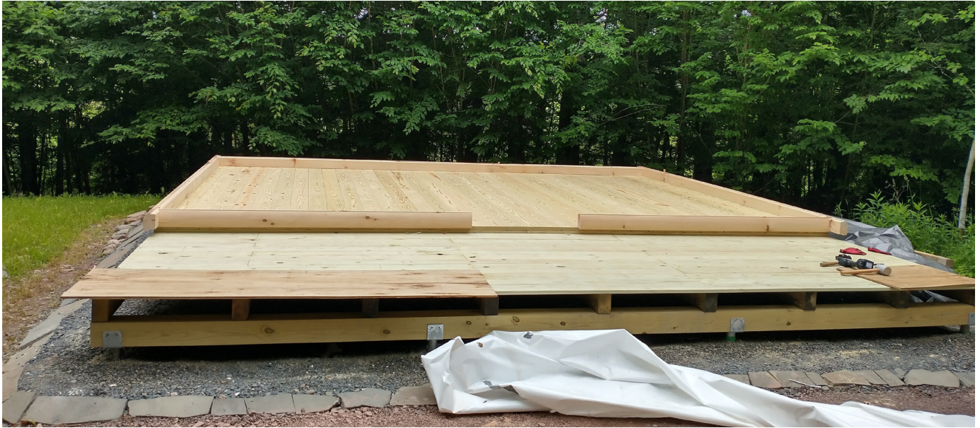
First row logs laid out and screwed in place
