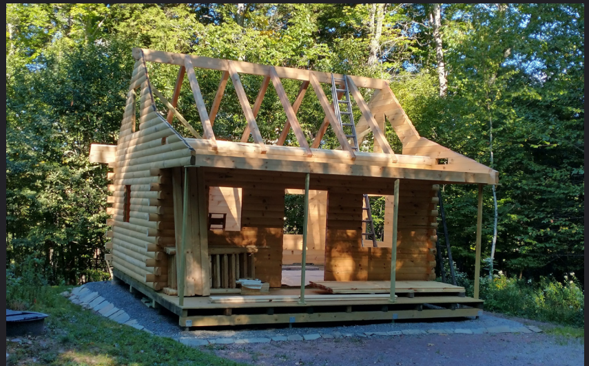
Fasten rafters with two 8" screws at top and two 8" screws at the bottom.
