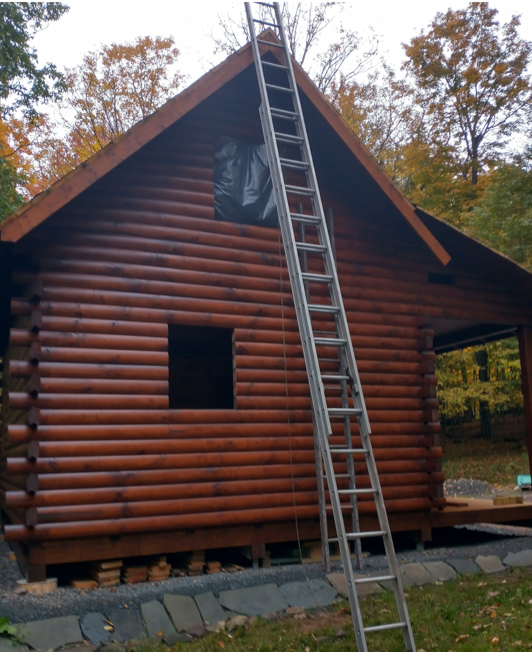
Pioneer style cabin: Some cutting will be needed to fit fascia at the transition.
