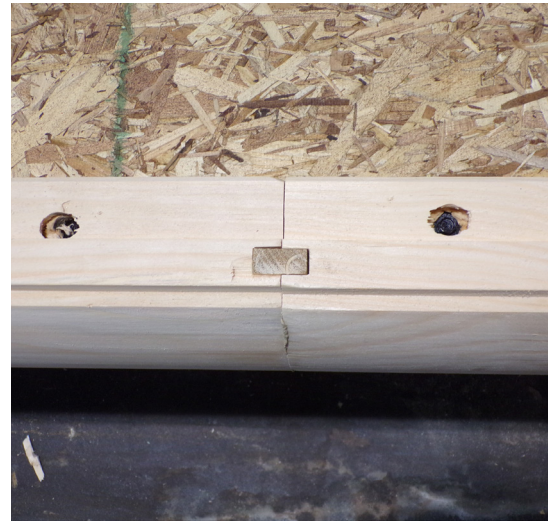
Caulk insert splice where butt joints come together and place screws on both sides of joint as pictured. Place screws every 3' along each row.
