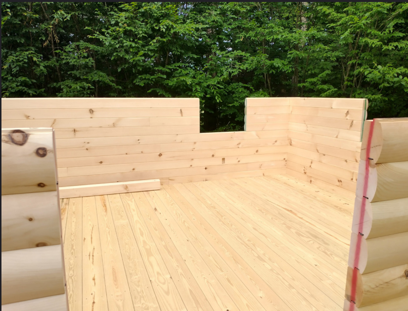
Color-coded ends help confirm location of each precut log along with numbers and letters.
