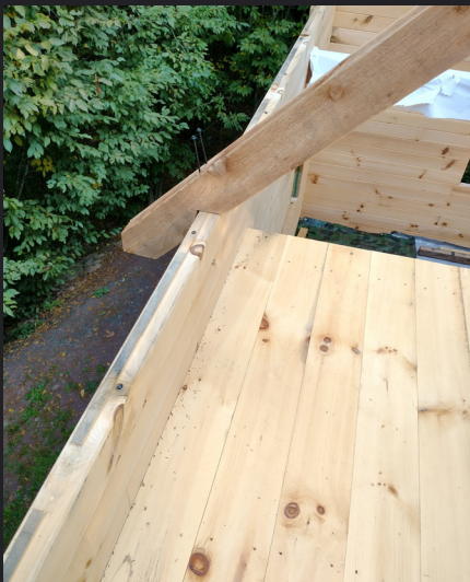
Installing loft gives you a working platform for installing beams and rafters.
