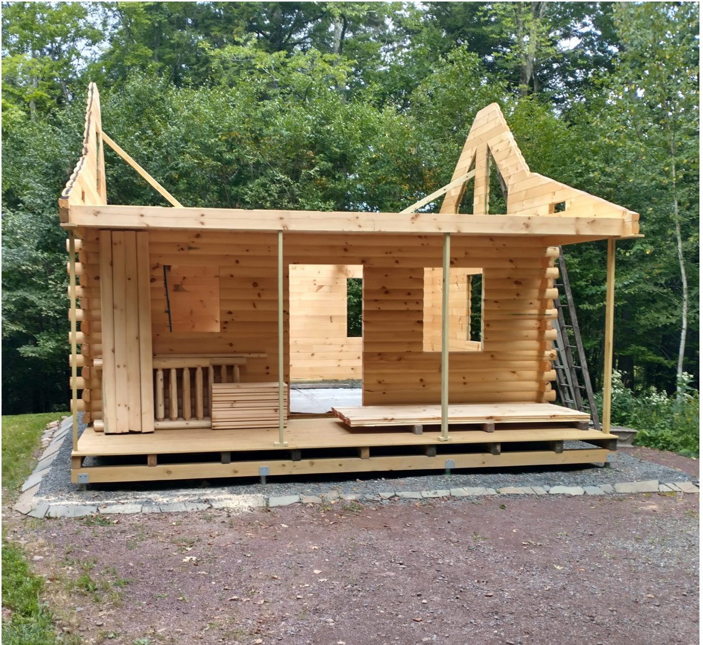
Brace gables before lifting ridge beam in place.
