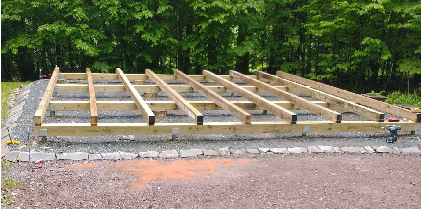
Concrete footer pads with brackets and 6x6 support beams. Gravel pad or concrete pad.
