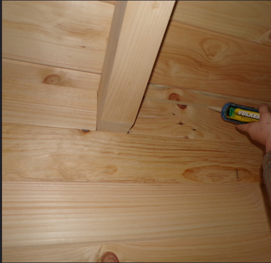
Caulk around perimeter of roof line to seal cabin.
